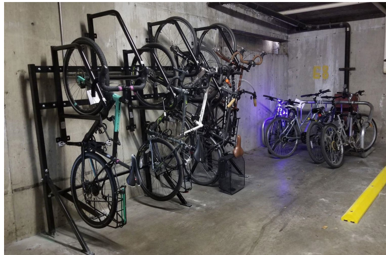
Bike Storage Racks
